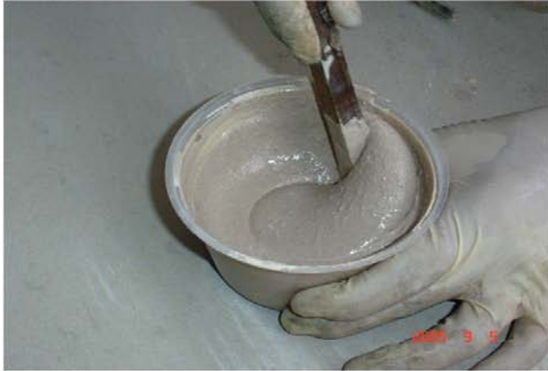
7. The mixture added with additives and hardener are mixed thoroughly.
